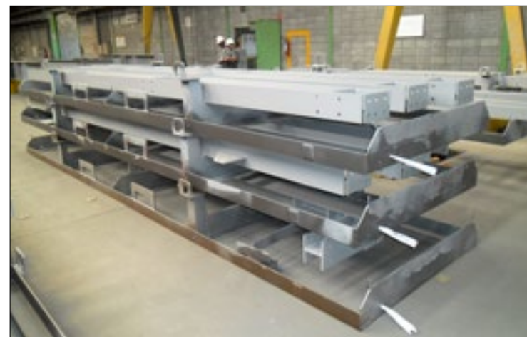
Racks de Pintura. Painting racks.
